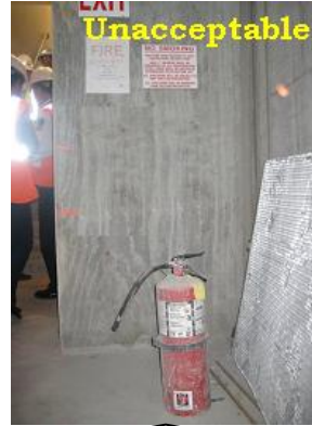
Improper floor placement of Fire Extinguisher.
