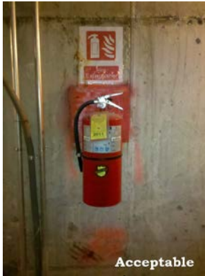
Fire extinguisher in a construction site.
